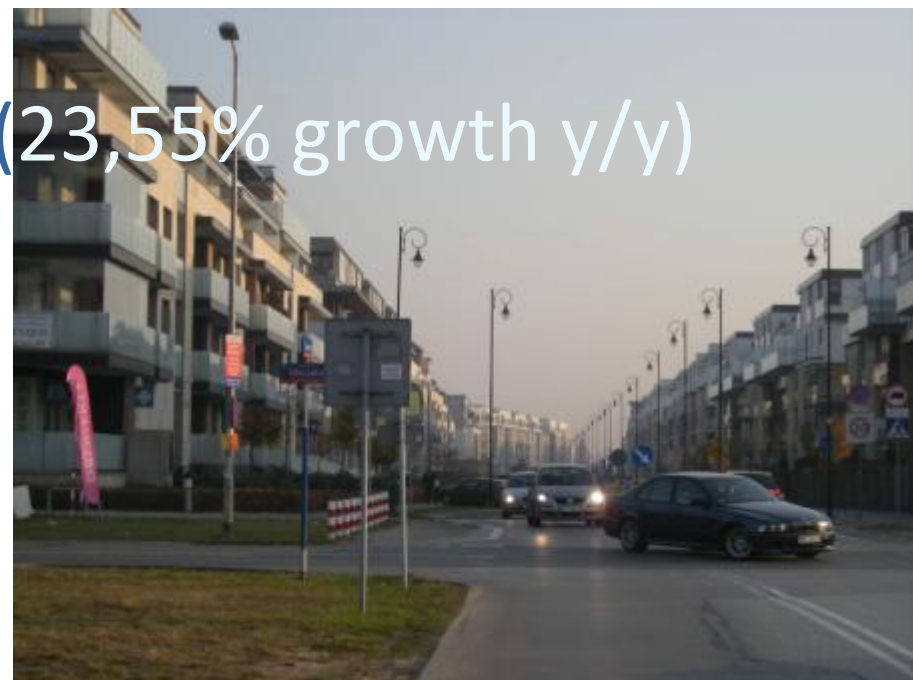
Construction of Miasteczko Wilanow in Warsaw
